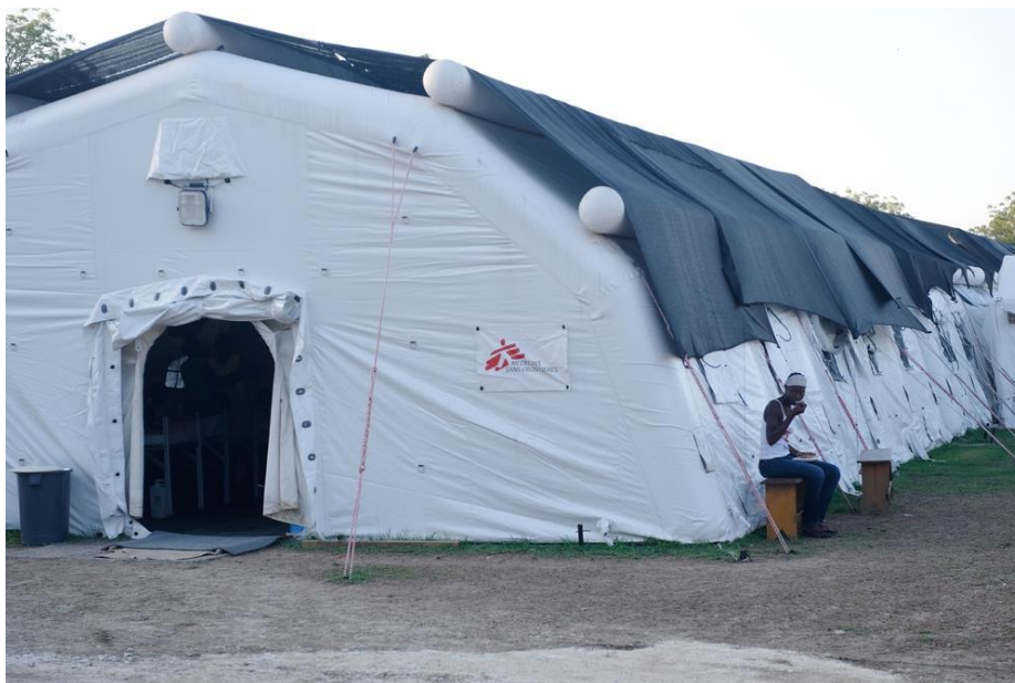
Figure 3.1 - An inflatable structure used by Medecins Sans Frontieres for a hospital after an earthquake in Haiti. Image credit www.doctorswithoutborders.org
